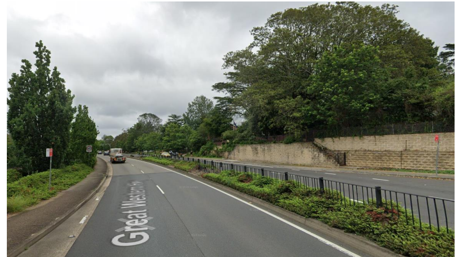
Figure 16 Planting along the Great Western Highway
