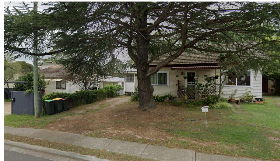
Figure 11 Weatherboard detached houses along the Great Western Highway
