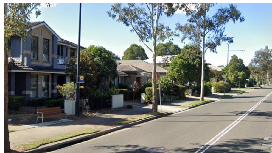
Figure 8 Example of bus stop infrastructure
