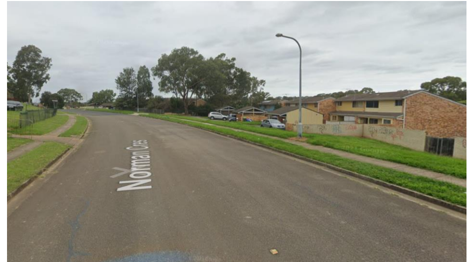
Figure 28 Footpaths on both sides of the local road
