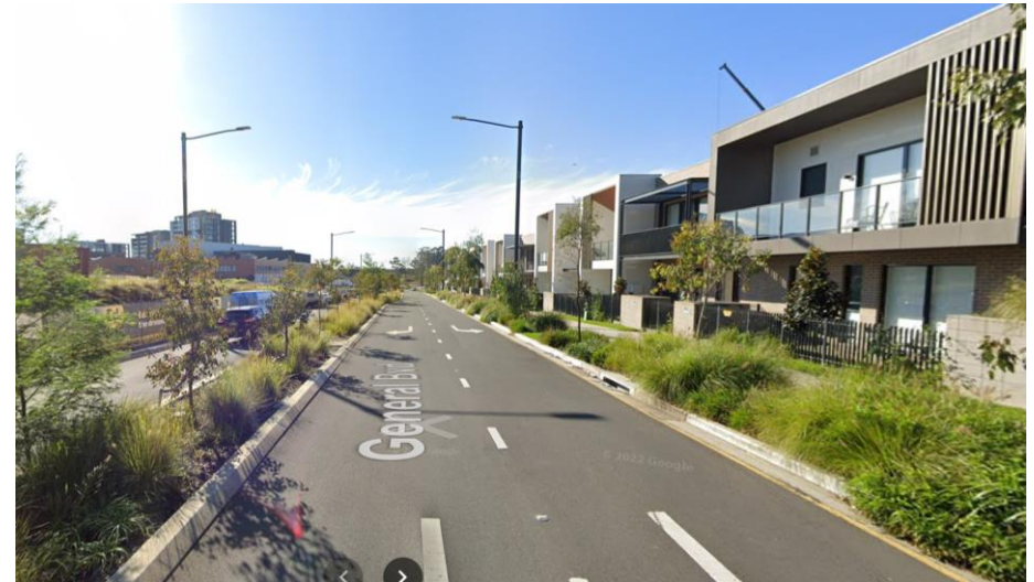
Figure 52 New street lights on residential streets
